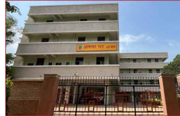
Contributed for construction of 2 out of 4 floors for Apna Ghar Ashram
