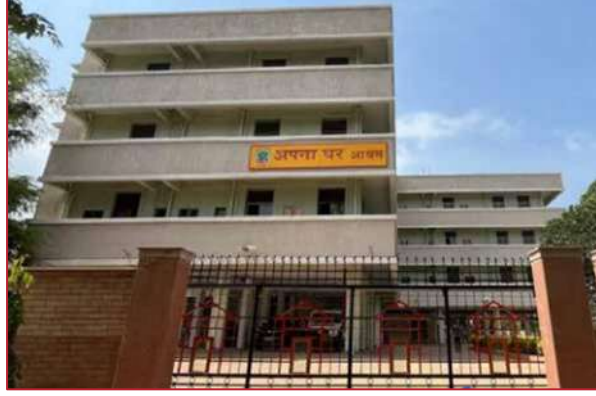
Contributed for construction of 2 out of 4 floors for Apna Ghar Ashram
