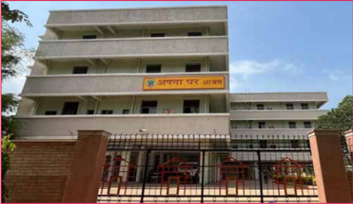
Contributed for construction of 2 out of 4 floors for Apna Ghar Ashram
